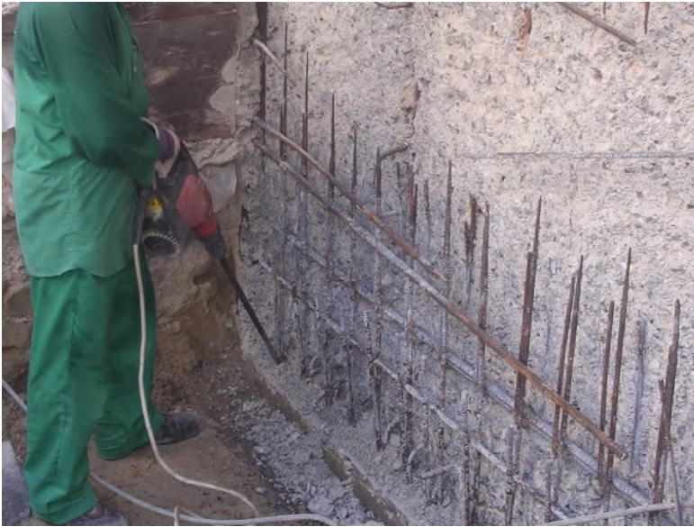
Figure 1 - Cleaning out behind the reinforcing
