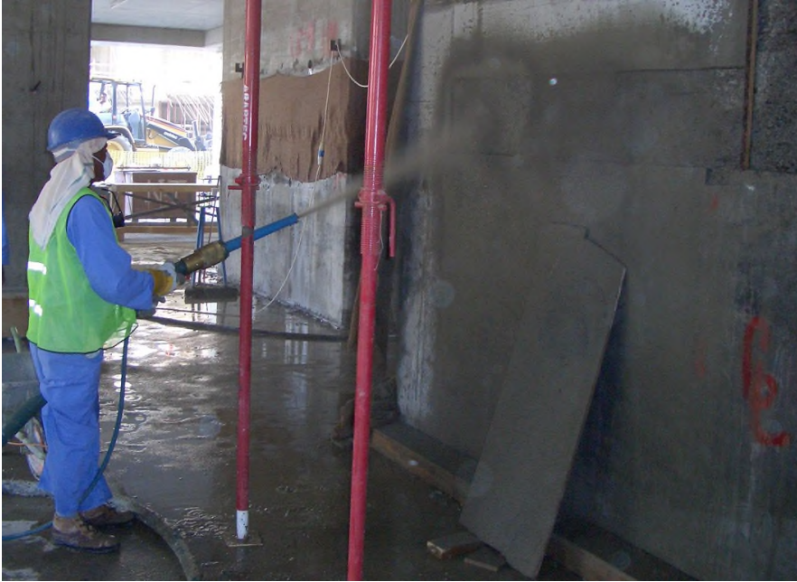
Figure 13 - Spraying on a wall
