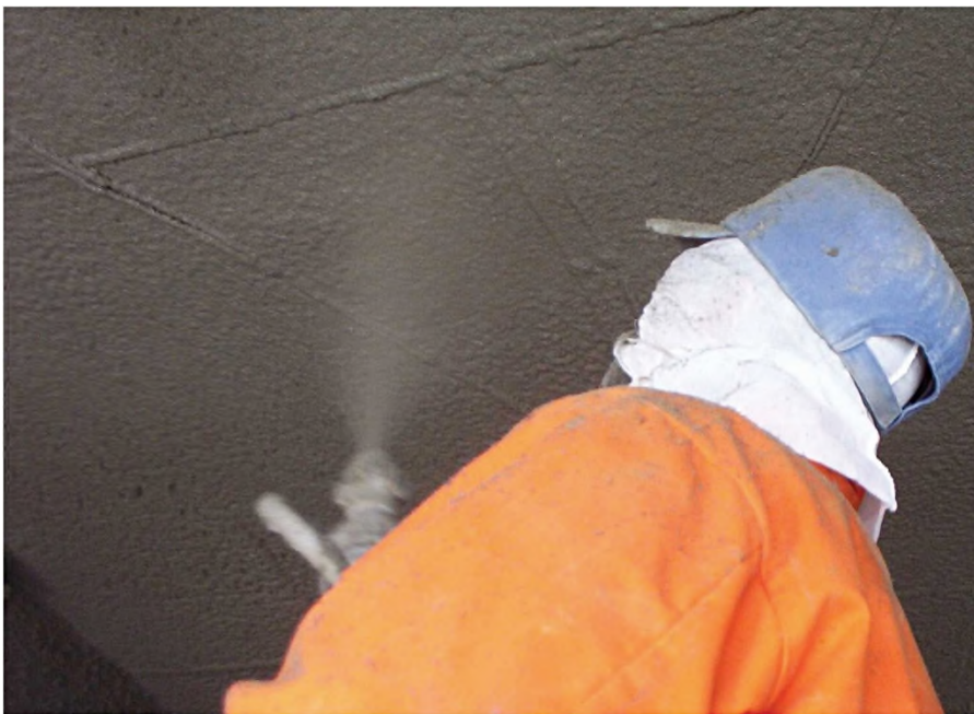
Figure 14 - Spraying mortar onto overhead repair
