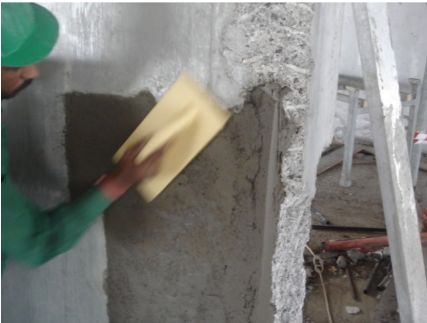
Figure 10 - Use a sponge float to get good surface
