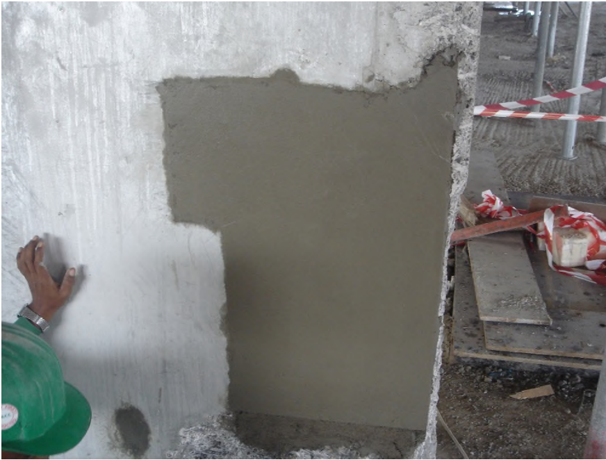
Figure 11 - Finished patch ready for curing
