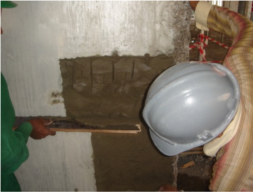
Figure 9 - Screed off to give flat surface
