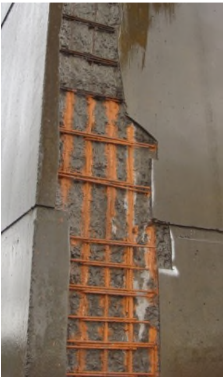
Figure 4 - Shows the MasterEmaco P 5000AP applied to prepared steel
