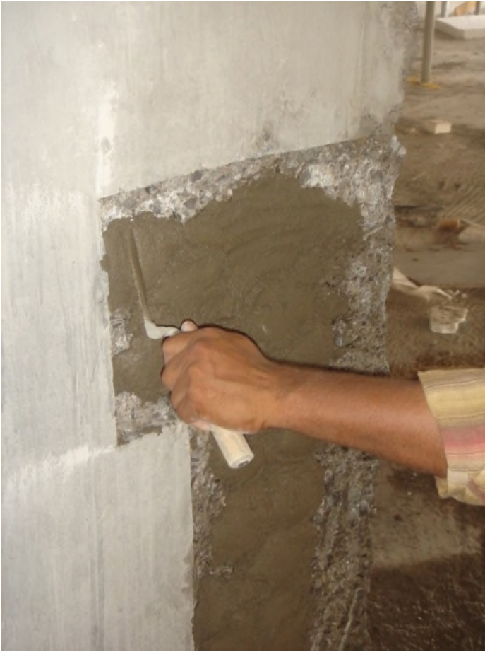
Figure 7 - Apply a slurry coat
