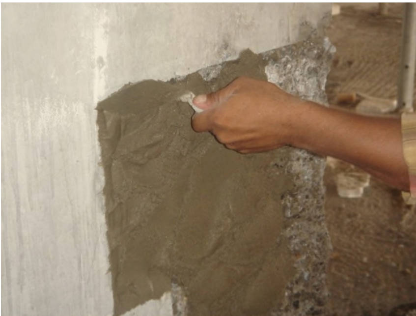
Figure 8 - Build up repair in layers
