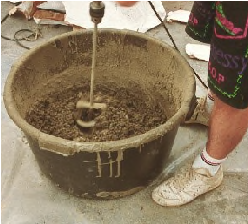
Figure 5 Mixing the repair mortar
