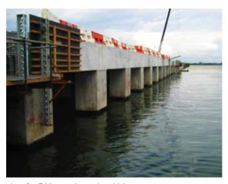
place for 24 hours. In marine tidal areas CSA cement grout may acceptably be submersed immediately in seawater without affecting the quality of the final product, as submersion in seawater actually improves its longterm strength. This is helpful for application to marine wharfs and seawalls, where work is completed at low tide.
